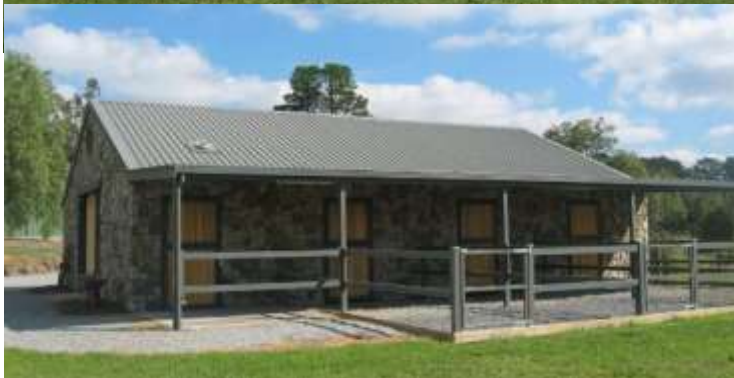
Stone veneer finish over full height concrete wall panels.
