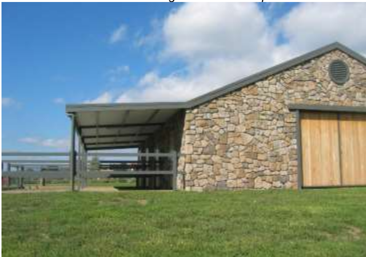
Stone veneer finish over full height concrete wall panels.
