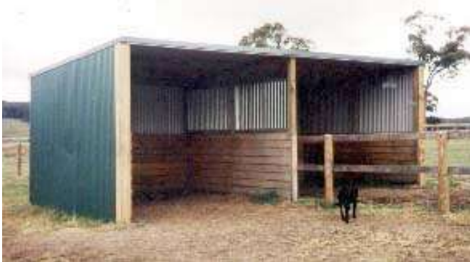
The timber shelter on the right has a 3.6m gate which is currently folded inwards so the shelter can be used as a walk in-walk-out shelter, but the gate can swing out (180 degrees) and then shut to contain the horse in the shelter. Gates can be added to shelters as required.
