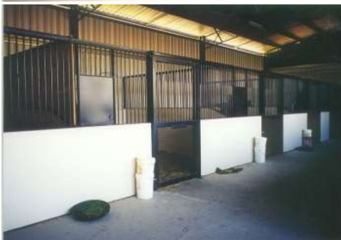
All concrete lower wall panels on this page.
